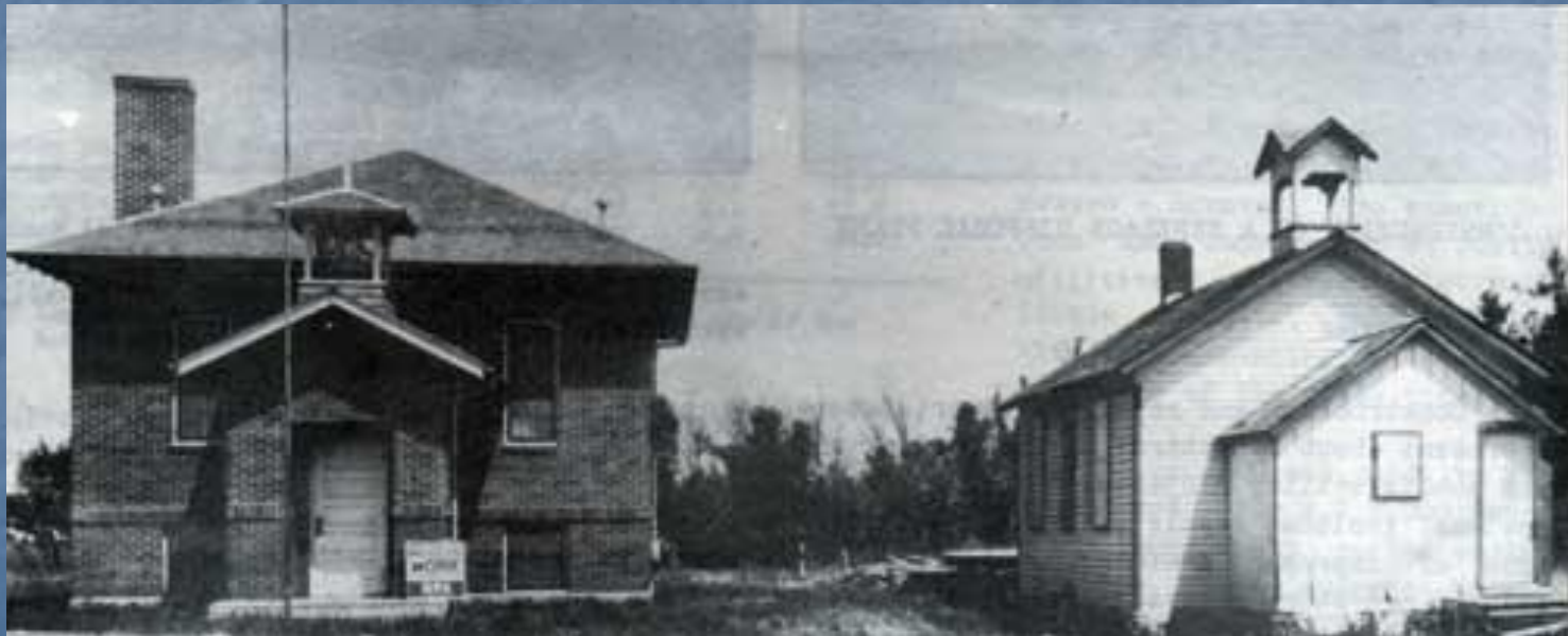
Building a new brick school to replace the older wooden one from 1876.
