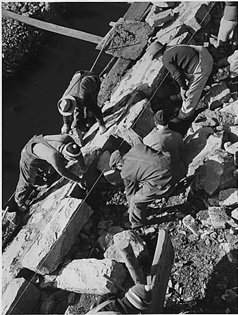
WPA roads project
